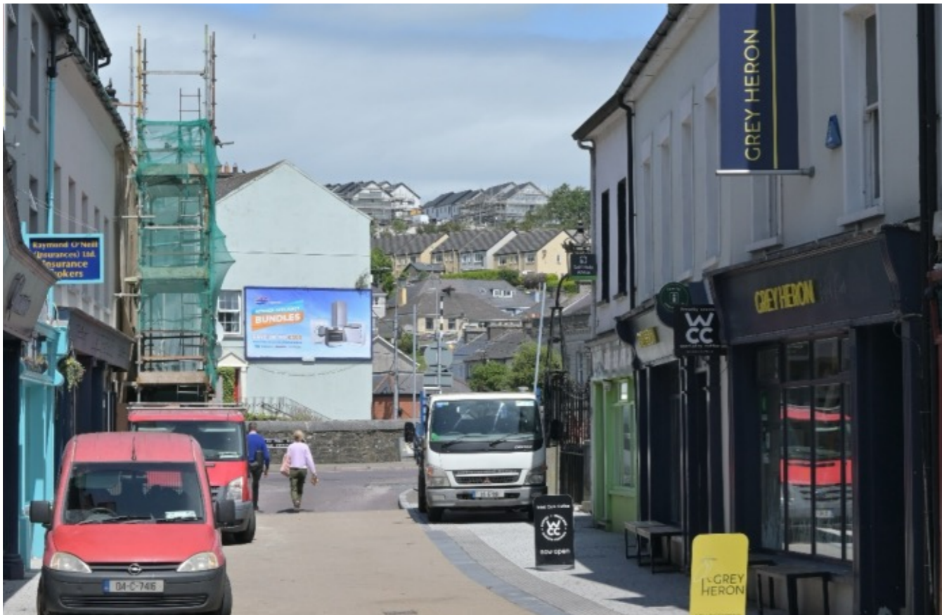
Figure 5-15 Housing under construction on Knockbrogan, visible from the town centre
