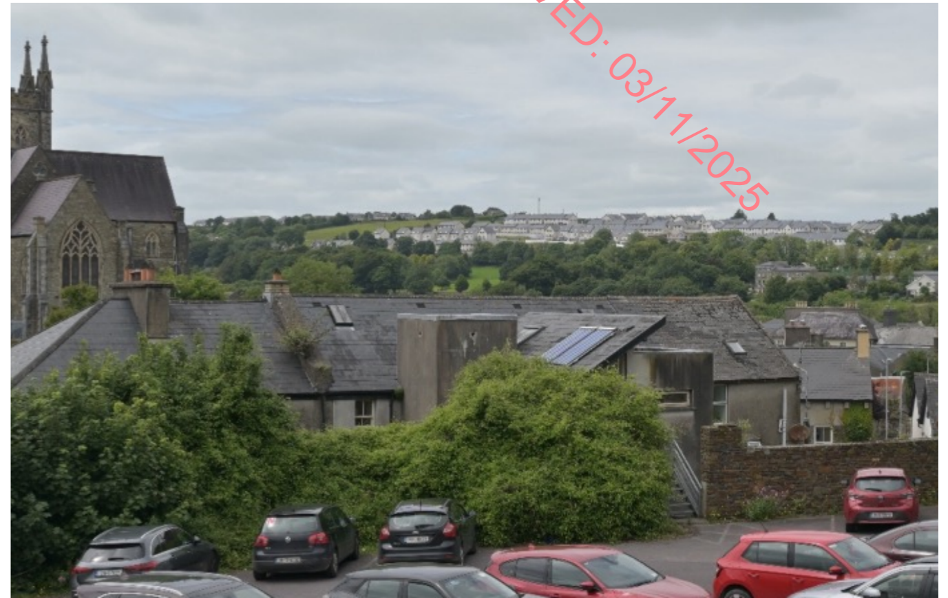
Figure 5-16 New housing off Upper Convent Hill to the north west of the town centre
